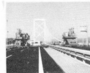
Vibrators at middle span
