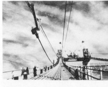
Erection of cable
