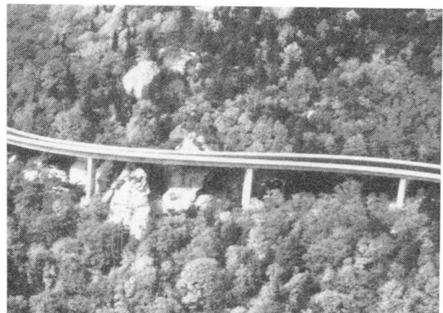
Fig. 6 - Harmonious integration of a highway in a National Park (USA)
