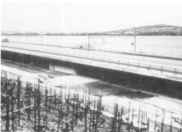
Fig. 5 - Highway on the border of the Bienna lake destroying the picturesque landscape (CH)
