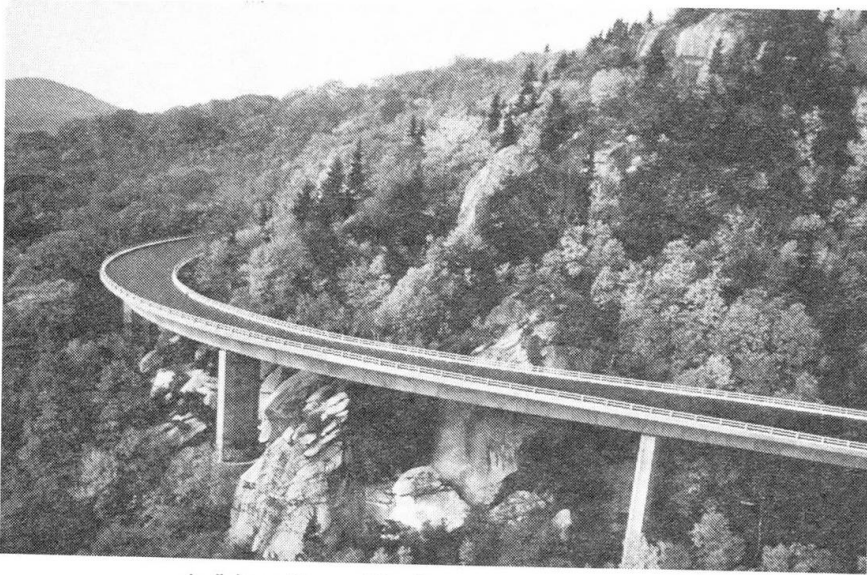
▲ Linn Cove Viaduct, NC ▶
