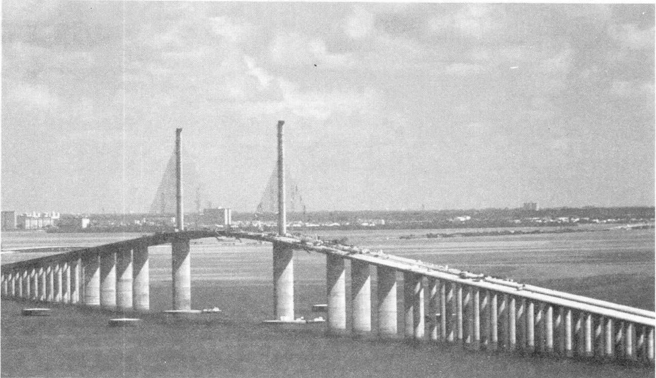
Fig. 11 Placing Last Segment in Main Span
