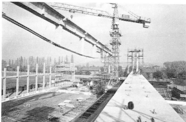
Fig. 1: Lifting of main beams
