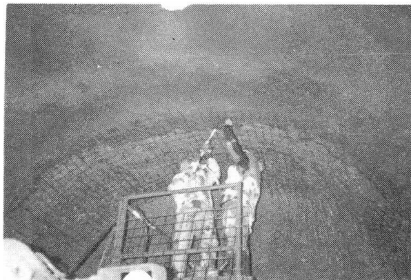
Fig.12 Reinforcing grids for shotcrete
