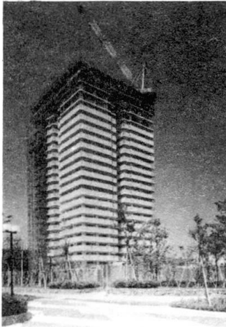
Fig.1 Building under construction
