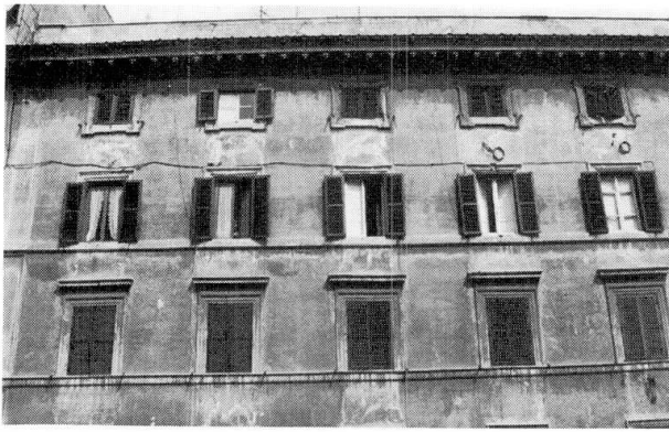
Fig. 12 Facade on Via Palestro with some of the installed instruments
