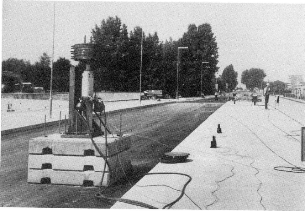
Fig. 3 Bridge Ulenbergstraße, hydraulic exciter (1st measurement)
