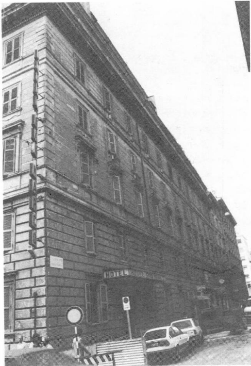
Fig. 3 Facade looking on Via Villafranca
