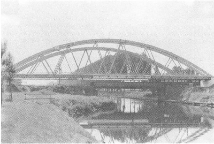
Photograph 1 Completed single-track bridge
