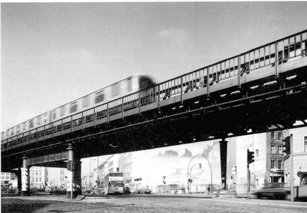
Figure 2. Truss girder bridge of the Berlin Underground, built in 1902, replaced in 1989
