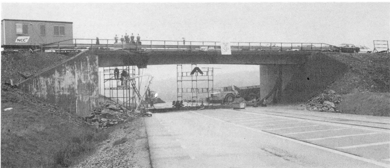
Fig. 4 View of the prestressed bridge
