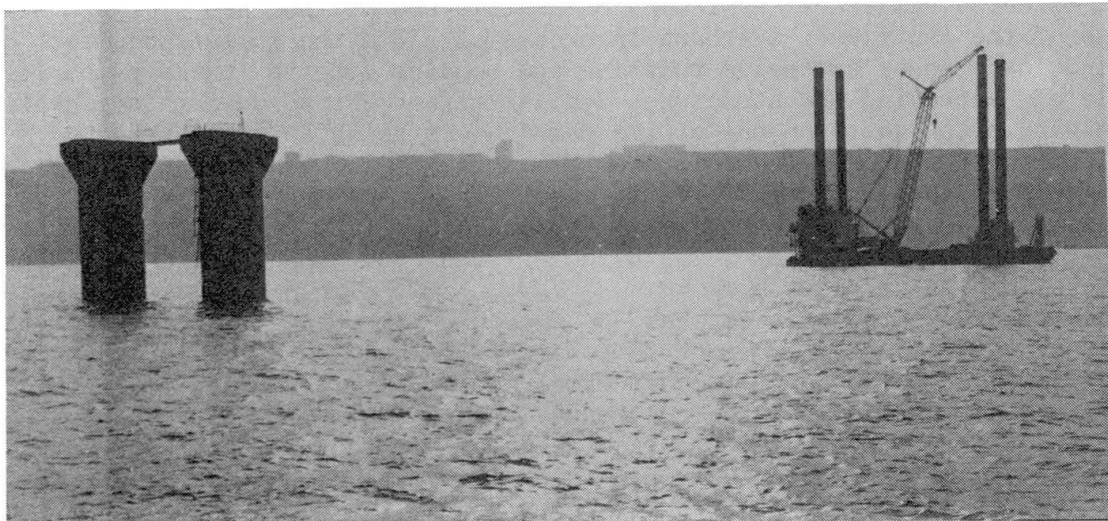
Fig. 5 Bridge bed pier
