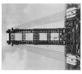
Photo 2 Side View of Temporary Cable-Stayed Tower
