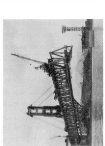
Photo 1 Full View of Steel Truss under Cantilever Erection
