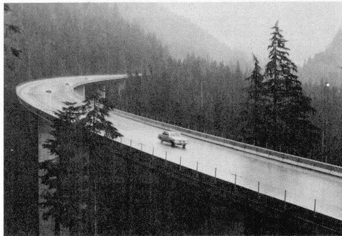
Fig. 13 Denny Creek Bridge Washington
