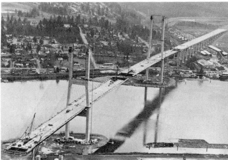
Fig. 6 Annacis Island Bridge Vancouver, B.C.
