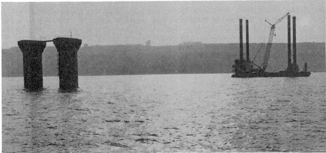
Fig. 5 Bridge bed pier
