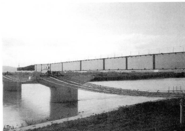
Fig.1 One stage of the launching erection method
