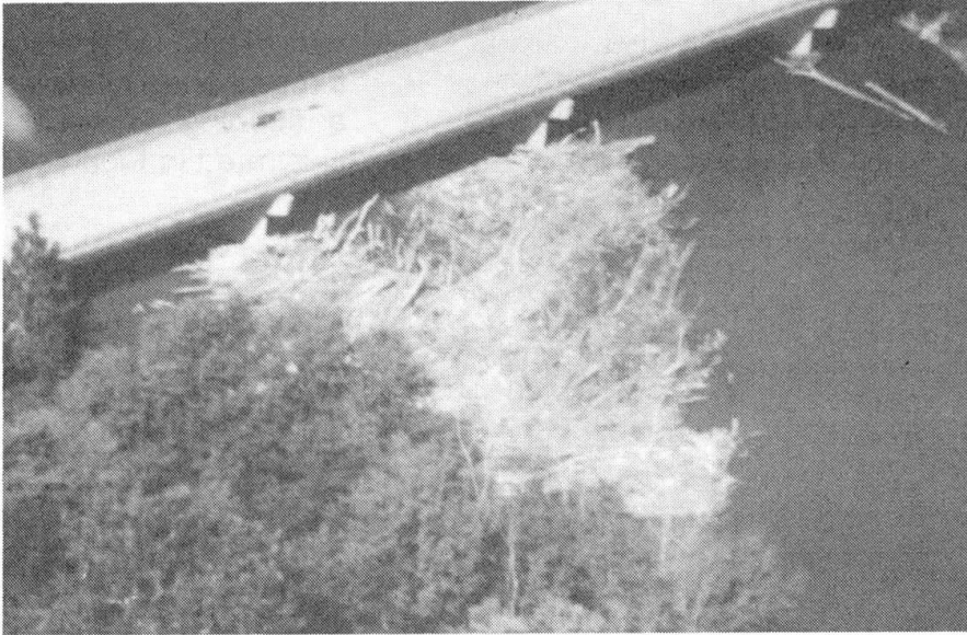
Figure 1. Typical Upstream Debris Accumulation
