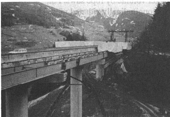
Fig. 9 Concreting at outer structure
