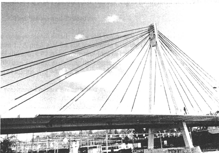
Figure 4: The cable-stay Stork bridge may be a milestone in bridge construction.
