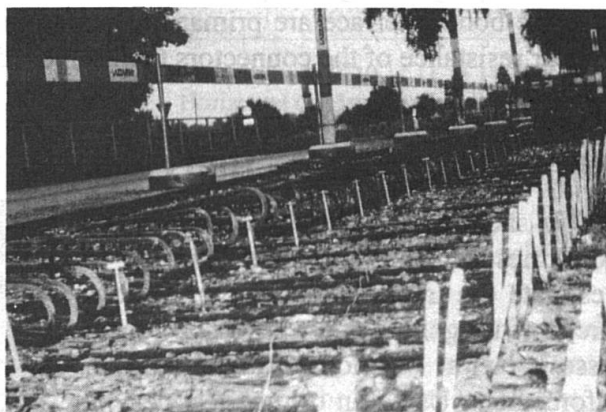
Fig. 1: Strengthening of a bridge
