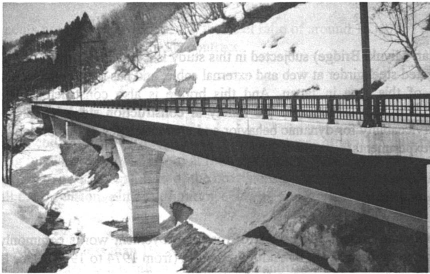
Photos-1 Side view of bridge
