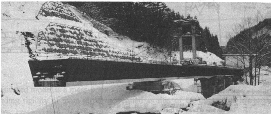
Photos-2 Incremental launching condition
