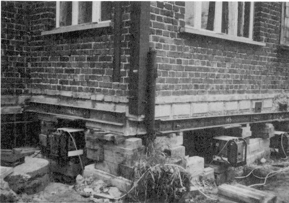
Fig.2 Built in jacks in cellar storey
