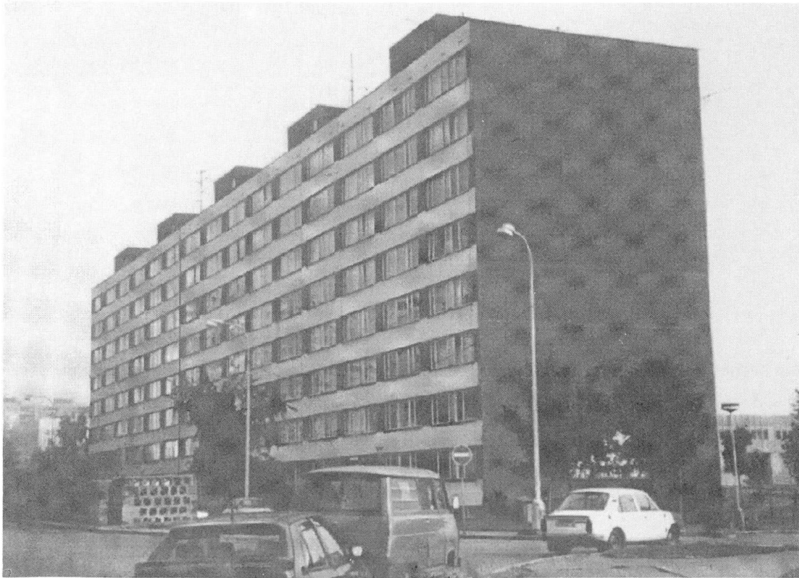
Fig. 1: Photograph of the tested panel building
