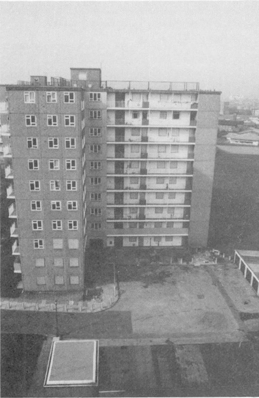
Fig. 1 External view of a Reema Conclad block
