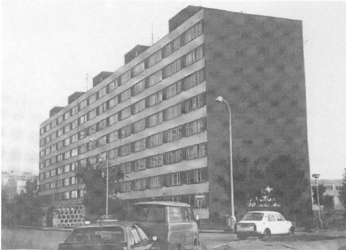
Fig. 1: Photograph of the tested panel building
