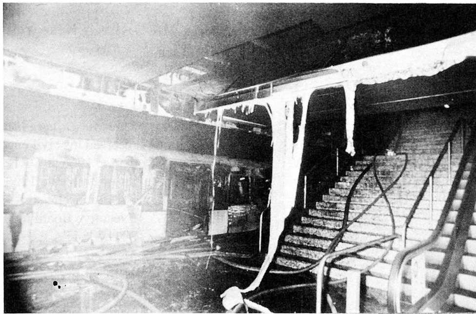
Fig. 1 Destroyed vehicles and interior furnishings at a stop following an urban commuter train fire on April 8, 1980 in Hamburg, Germany
