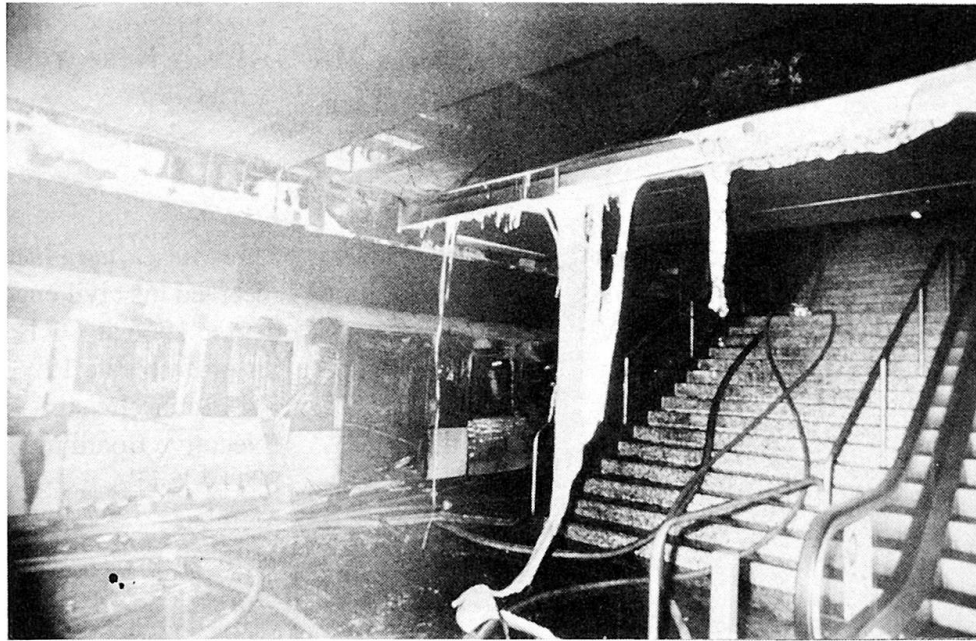
Fig. 1 Destroyed vehicles and interior furnishings at a stop following an urban commuter train fire on April 8, 1980 in Hamburg, Germany
