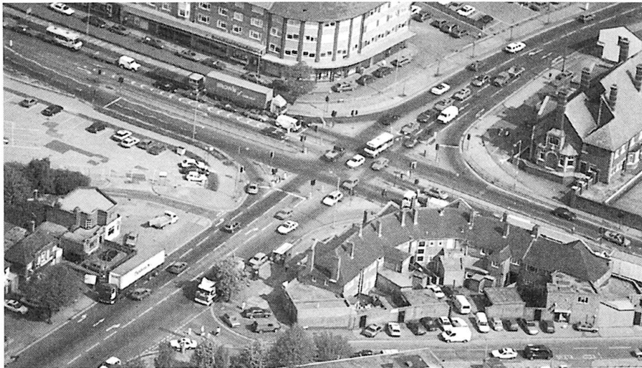
Figure 1: Meir Crossroads prior to construction
