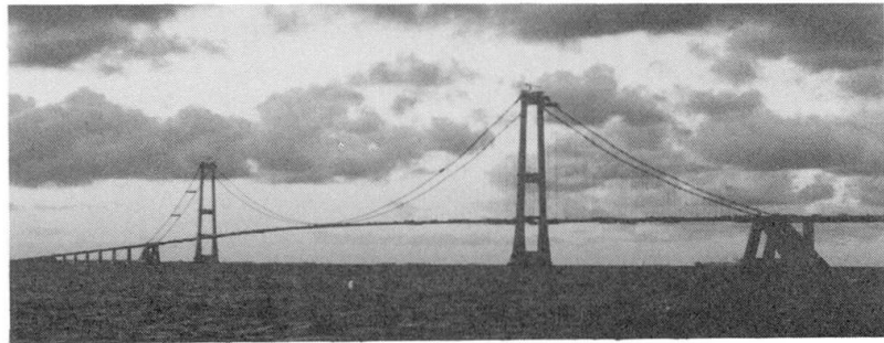
Fig. 1 - 2 - Before and after the erection work
