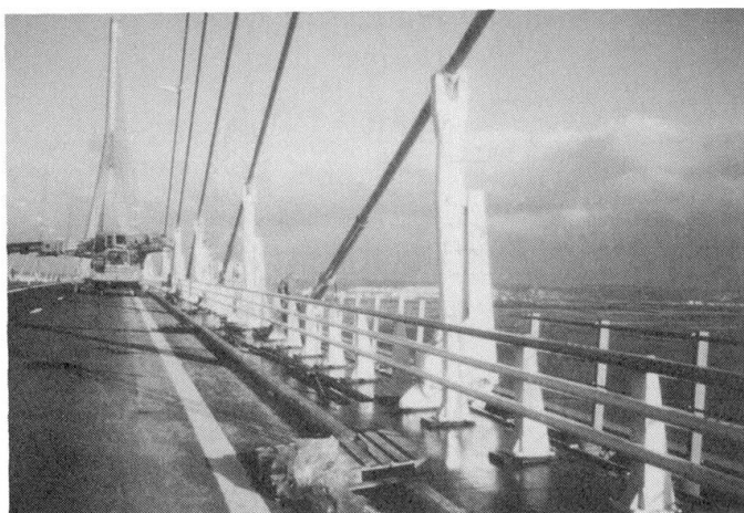
Normandie Bridge : Damping ropes and hydraulic dampers
