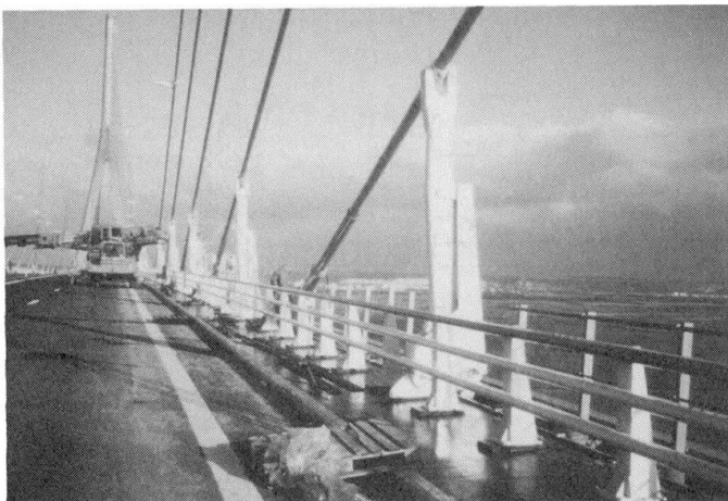
Normandie Bridge : Damping ropes and hydraulic dampers
