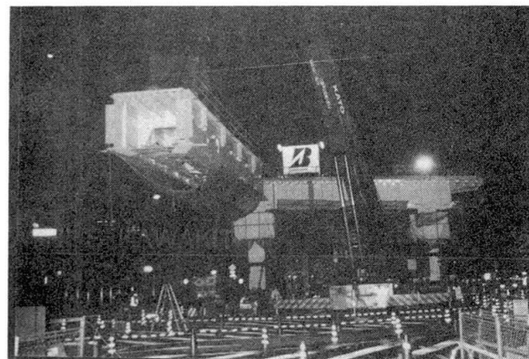
Photo. 3 Erection of Girder and Deck
