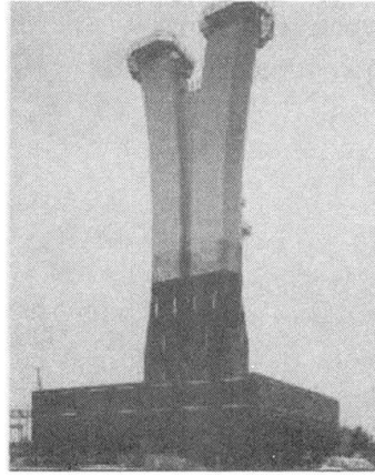
Fig. 2 Steel pier of Trans-Tokyo Bay Bridge
