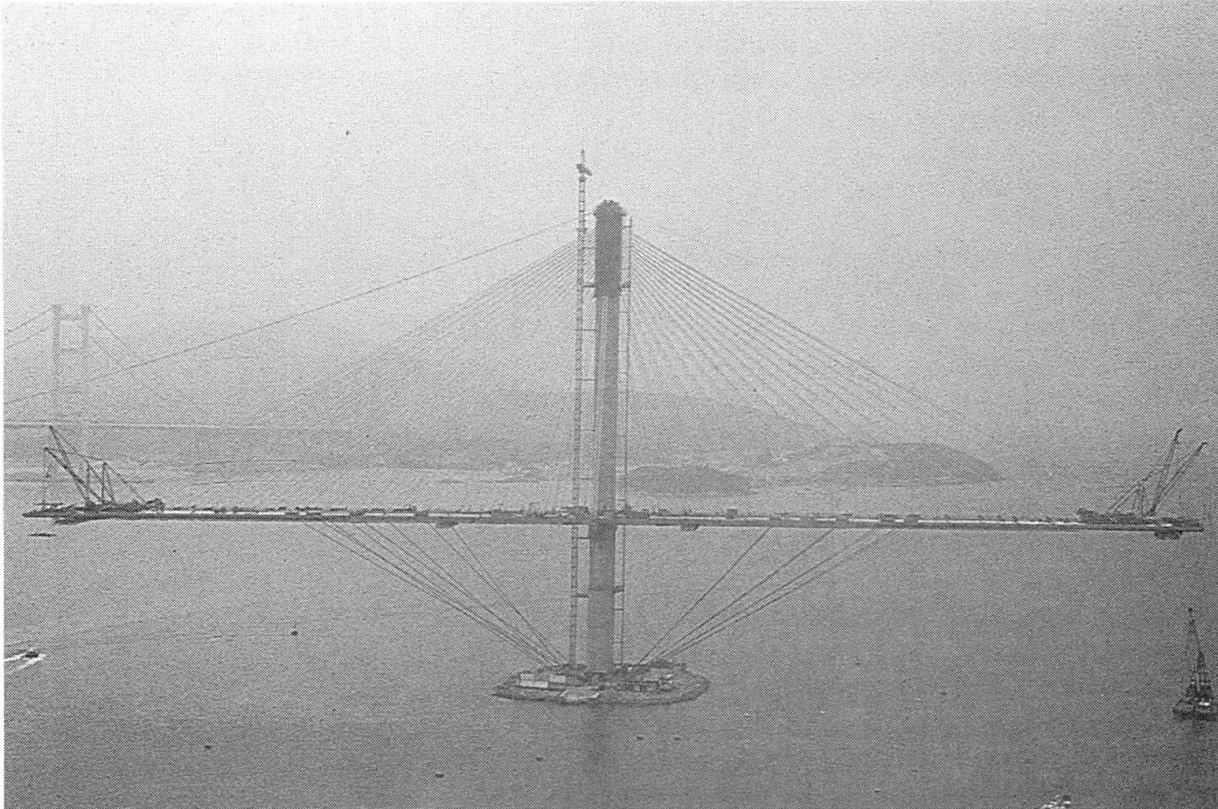
Fig. 6 Main cantilever
