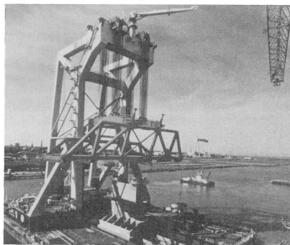
Fig. 9 First pier at load-out jetty
