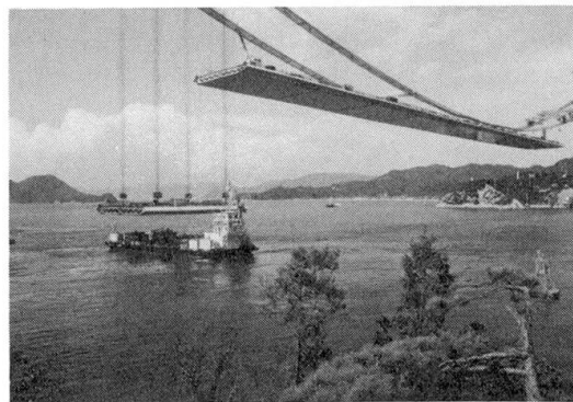
Fig.4 View of the girder erection
