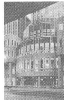
26 The base of North West Tower
