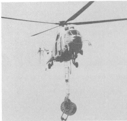
Photo.2 Carrying a pilot rope by helicopter
