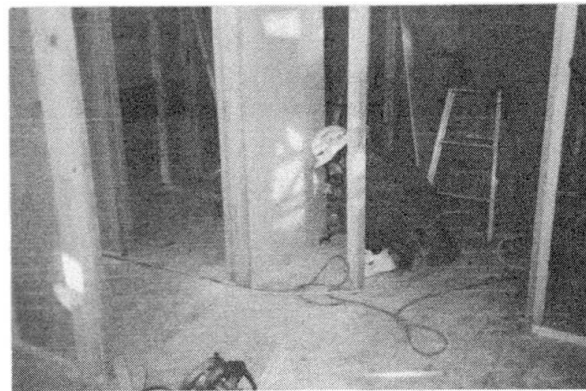
Fig. 2 Installation of half-panel parts
