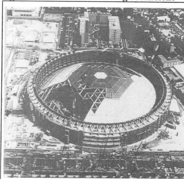
Photo. 3-1 Over view of construction state
