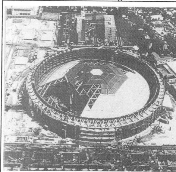
Photo. 3-1 Over view of construction state
