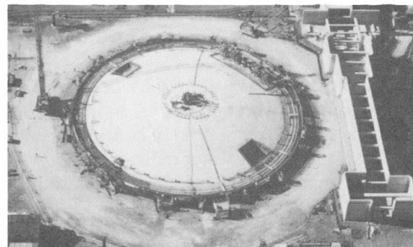
Fig. 11 Over-view of concrete dome roof
