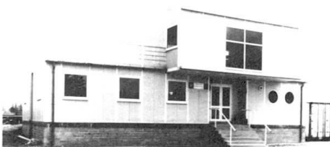
Fig. 7 Second Severn Crossing site office
