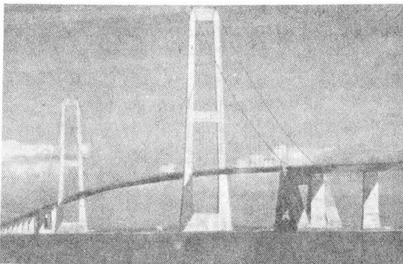
The East Bridge.
