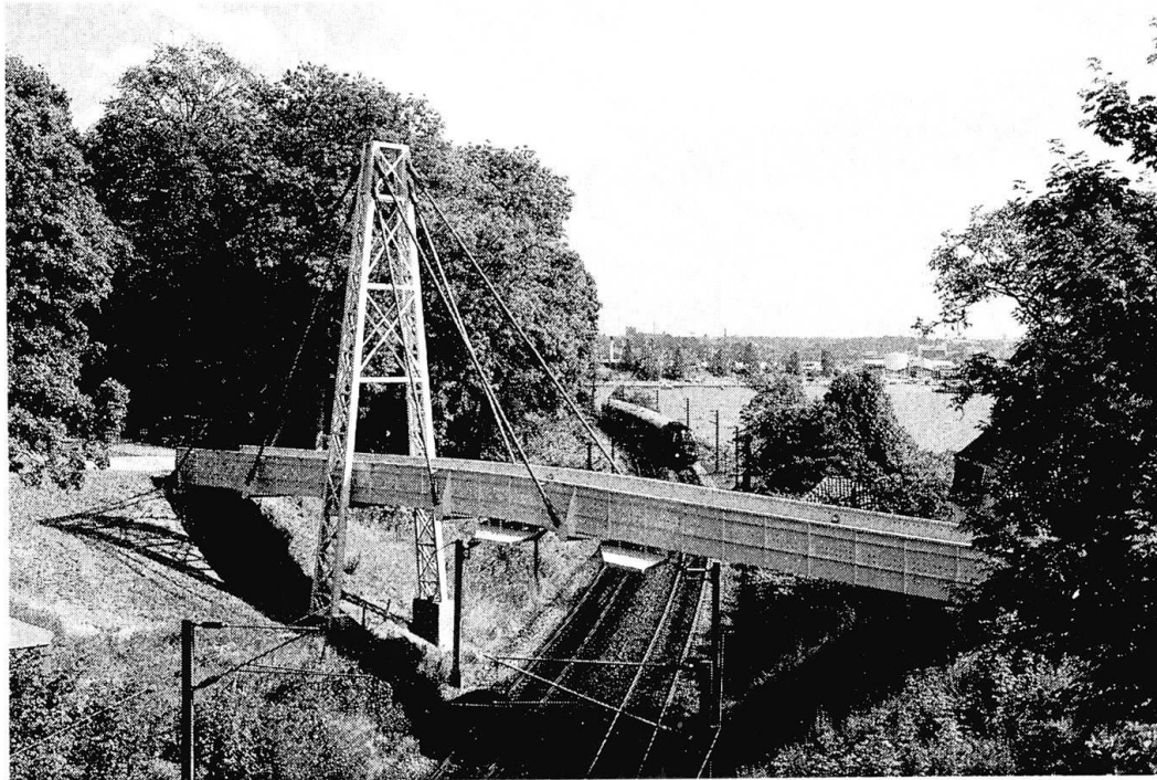
Fig. 1. Fiberline Bridge at Kolding, Denmark
