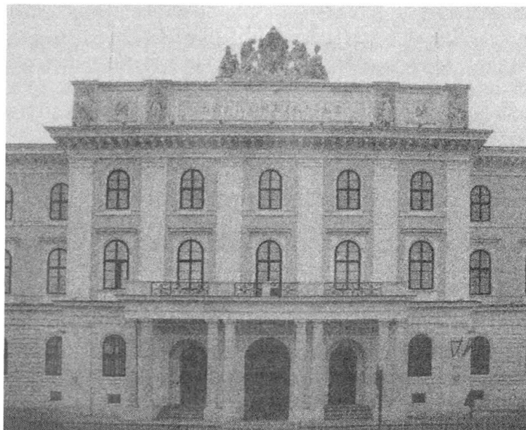
Fig. 1: Aspect of the renovated and strengthened edifice from the main road "Am Heumarkt 1"
