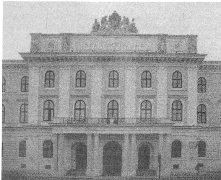
Fig. 1: Aspect of the renovated and strengthened edifice from the main road "Am Heumarkt 1"
