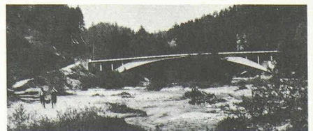
2051 Schwarzenburg 1932 Rossgrabenbrücke, Ing. Maillart Robert
