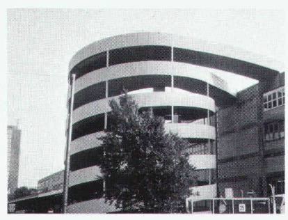
Rampe de parking Migros Herdern
