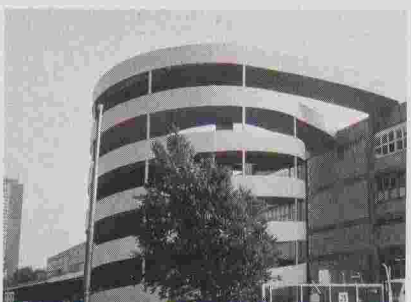
Rampe de parking Migros Herdern
