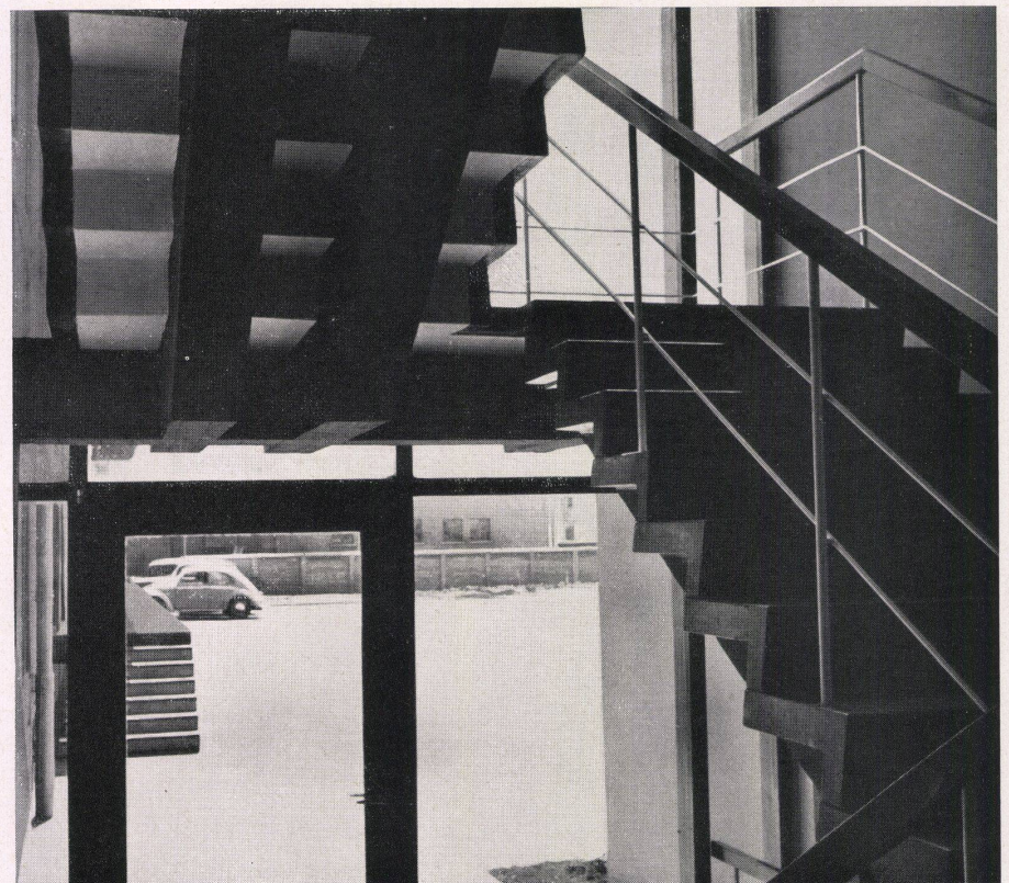
Staircase between administration building and warehouse.
