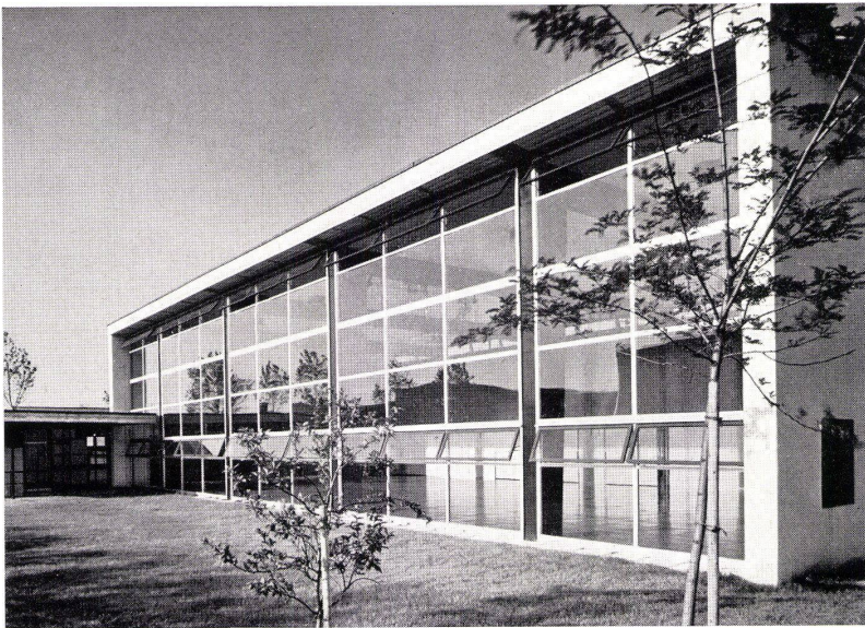
Turnhalle Wasgenring, Basel
